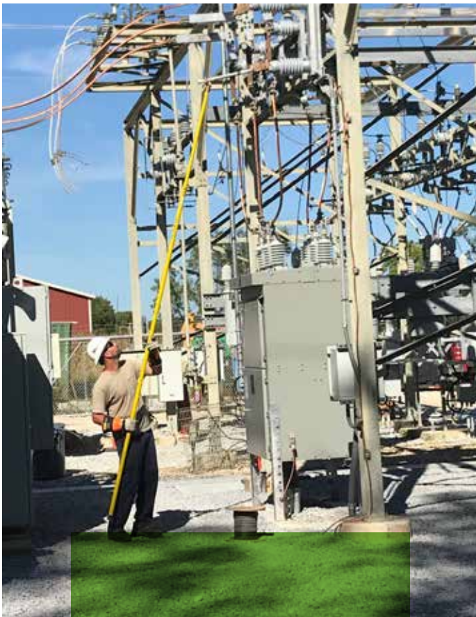
Journeyman First Class Brandon Beard flips the switch to bring one of the new transformers online at the Fairfield Substation.
